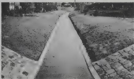
A well-designed storm drain in Fairfax, Virginia, has a semi-fixed liner to drain away erosive storm water. —Journal of Soil and Water Conservation
